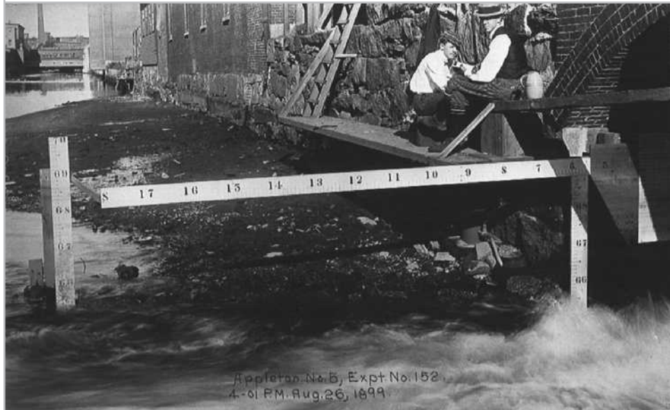
FIGURE 1-2 THE CITY OF LOWELL, MASSACHUSETTS, WAS THE SITE OF A FAMOUS SERIES OF WATER POWER EXPERIMENTS CONDUCTED BY JAMES FRANCIS AND URIAH BOYDEN. THE PUBLICATION OF THE RESULTS IN 1855 CONTRIBUTED GREATLY TO THE FIELD OF HYDRAULIC ENGINEERING. HERE, TWO ASSISTANTS ARE SHOWN MEASURING WATER LEVELS.
